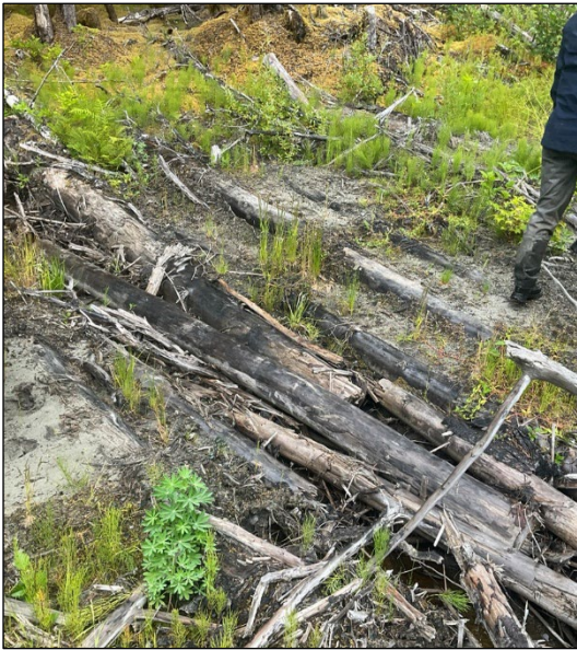
Figure 3.—Puncheon across the road at waypoint 762.
