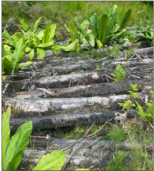
Figure 4.—Puncheon across the road at waypoint 764.
